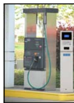
FF814 Card Reader Controller at Retail DTE CNG sites. Credit Cards and Receipts.
